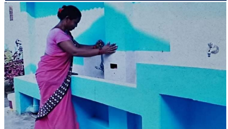
CARETAKER REPAIRING TAP
