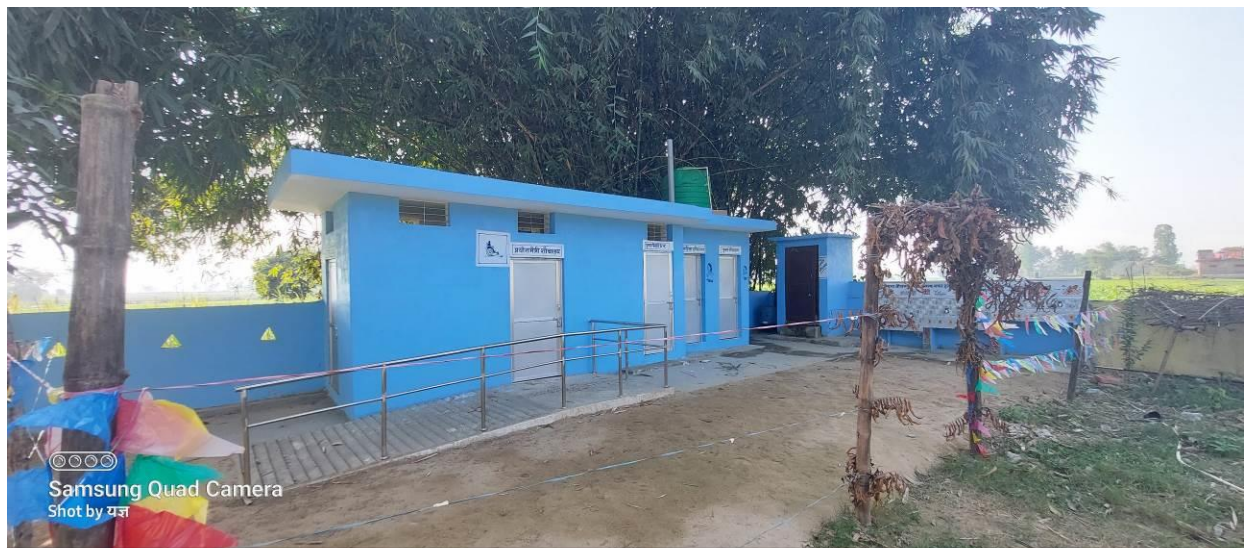
Parsauna Health Post/Birthing Center, Parsauna, Kolhabi-6, Bara
