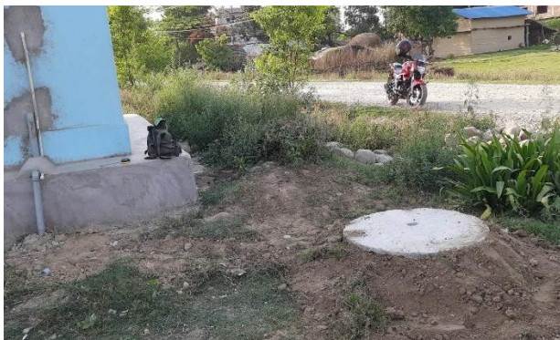
Constructed soak pits in in the ICs for the purpose of waste-water management
