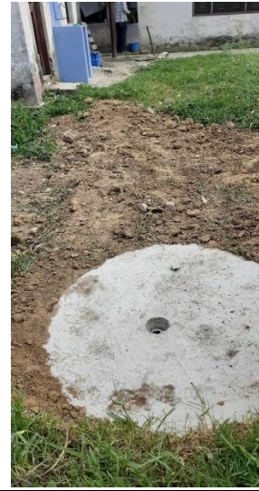
Construction of soakpits and realigning pipe line route to sort the identified problems during visit
