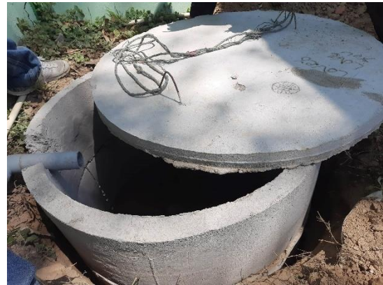
Constructed soak pits in in the ICs for the purpose of waste-water management
