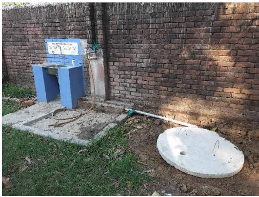
Construction of soakpits and realigning pipe line route to sort the identified problems during visit
