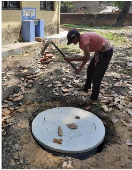
Construction of soakpits and realigning pipe line route to sort the identified problems during visit
